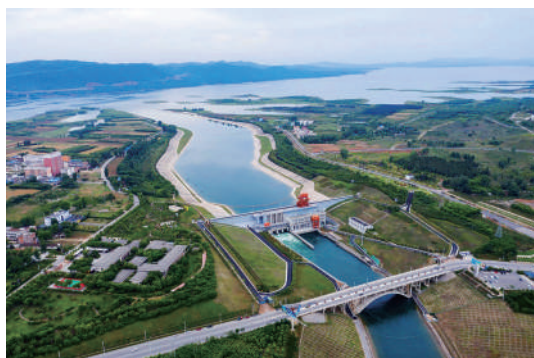
The Taocha Canal Head of the Central Route of the South-to-North Water Diversion Project in Xichuan County, Nanyang City, Henan Province. (Drone photo taken on May 20, 2021, by Cai Yang, Xinhua News Agency.)
