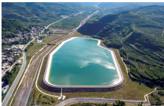
Yangjiawan storage facility of the Taohe River water diversion project in Tianshui, Gansu Province. (Drone photo taken on September 8, 2021, by Fan Peishen, Xinhua News Agency.)
