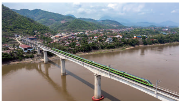
A China-Laos Railway passenger train runs on the Mekong River Bridge in Luang Prabang, Laos, May 28, 2023. (Drone Photo) Xinhua/Chen Chang
