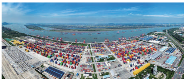
A view of the container terminal at bustling Longtan Port Area, Nanjing Port. (Panoramic drone photo taken on September 25, 2024, by Li Bo, Xinhua News Agency.)
