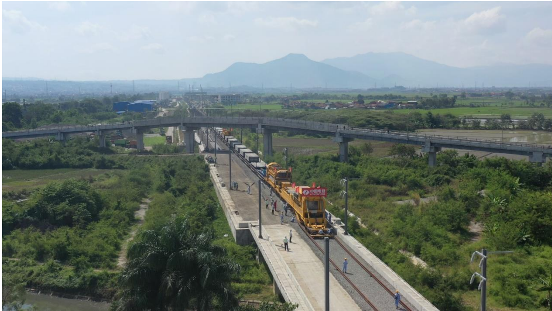
Photo taken by a drone in Bandung, Indonesia on July 1, 2022 shows the construction site of ballast track laying on the main line of the Jakarta-Bandung High-Speed Railway. (Xinhua/Yu Zhongbao)
